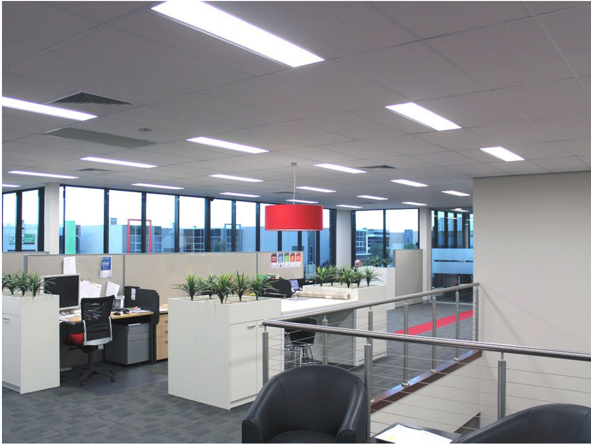
Image 5.4 – A SMD-fixture lighting application of an office building.
